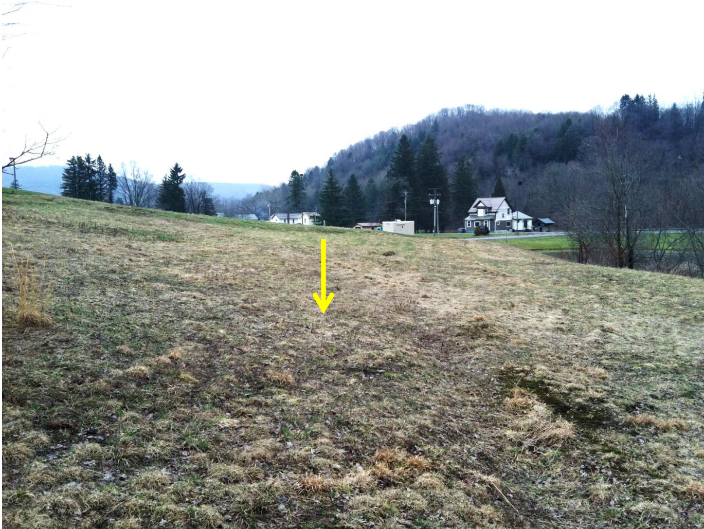
PHOTO 5: BIO-RETENTION AREA (150-FT x 50-FT) LOCATED ON A NATURAL “SHELF” ABOVE AND TO THE NORTH OF THE STORMWATER POND.
