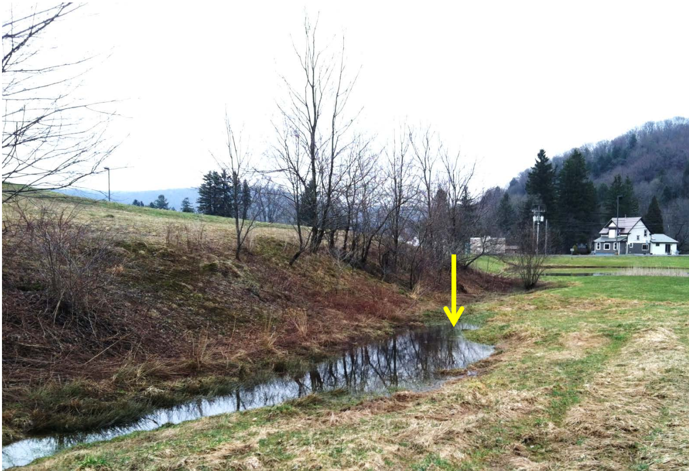
PHOTO 4: CONSTRUCTED WETLAND (150-FT LONG x 10-30-FT WIDE) LOCATED WEST OF THE STORMWATER POND. NOTE THAT THE BIO-RETENTION AREA WILL BE LOCATED ON THE NATURAL “SHELF” ABOVE THE WETLAND (SEE PHOTO 5).
