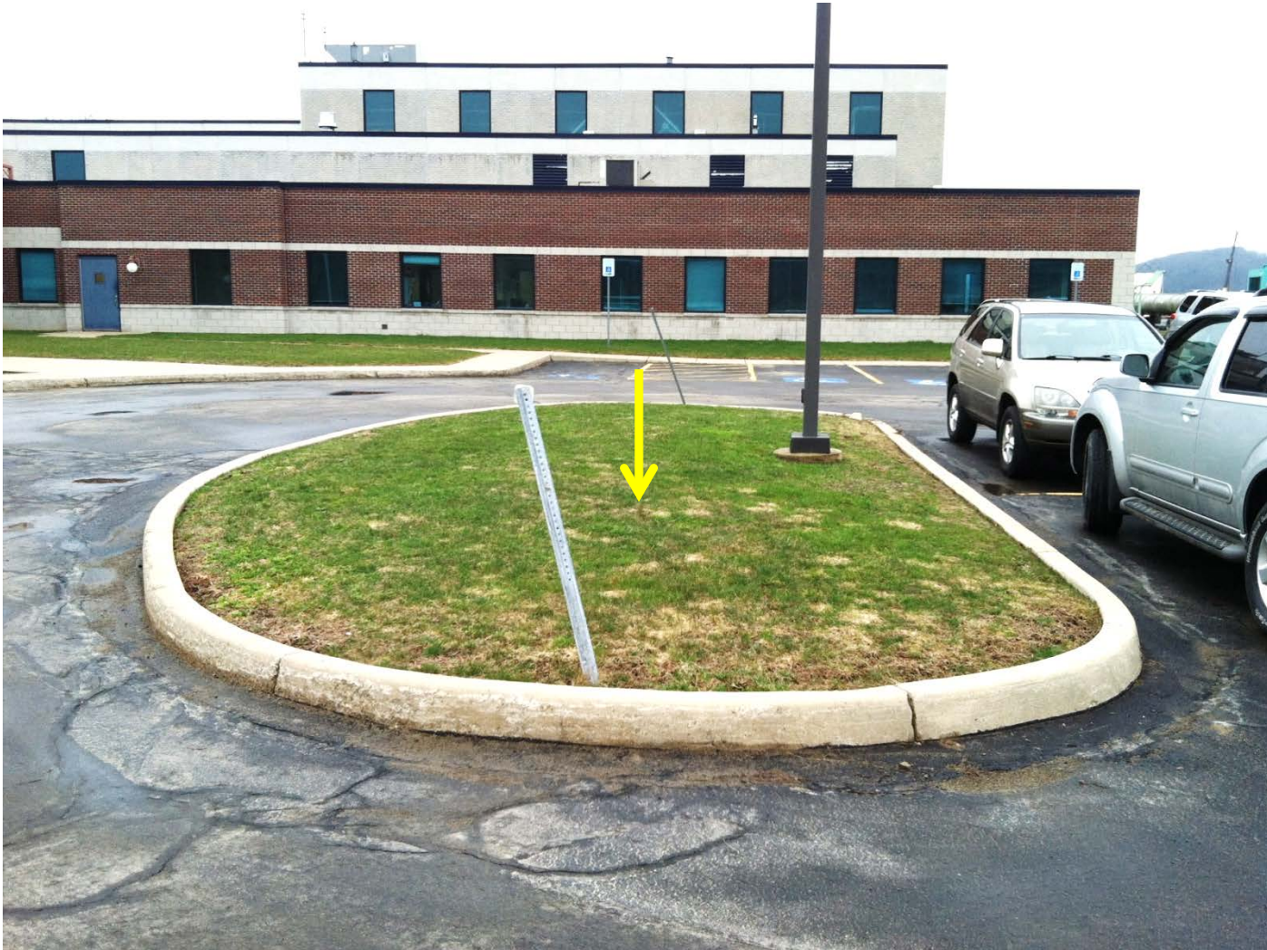
PHOTO 1: INFILTRATION GARDEN (400-FT 2 ) LOCATED AT THE WEST END OF PARKING LOT.
