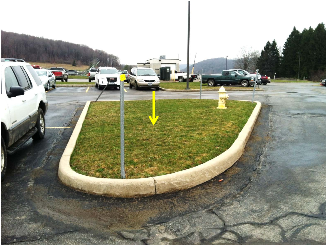
PHOTO 2: INFILTRATION GARDEN (400-FT 2 ) LOCATED AT THE EAST END OF PARKING LOT.
