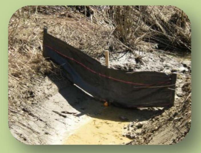
WRONG! An example of an ineffective erosion control practice – silt fencing should be buried to a depth of about 8 inches and should not be used in drainage ways
