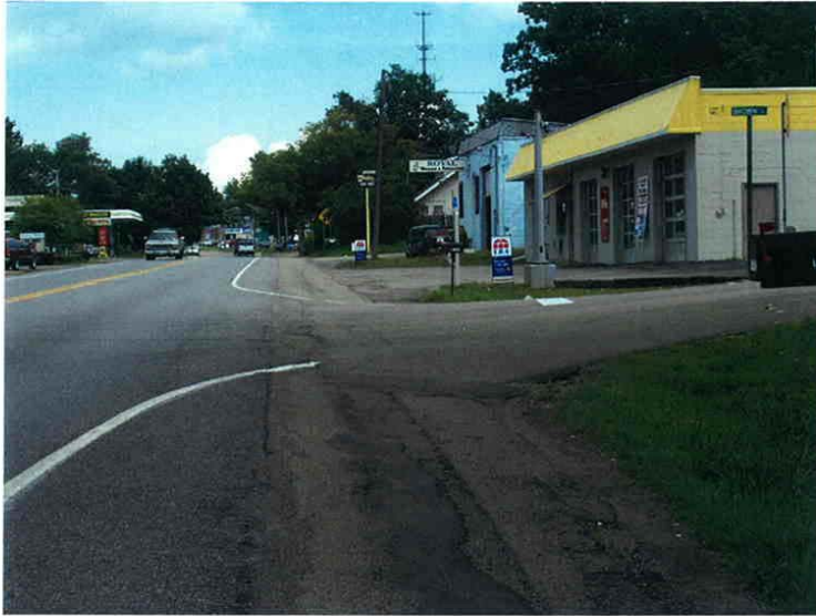
Photograph 7 Looking north on NYS Rt. 60, at the intersection of Brown Street, 2.0 miles north of the intersection with NYS Rt. 62. There are two 11.5' and 6' wide paved shoulders.
