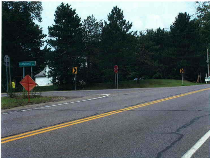
Photograph 6 Looking north on NYS Rt. 60, at the intersection of CR 49 (Kiantone Road). There are two 11.5' wide lanes and 5' wide paved shoulders.
