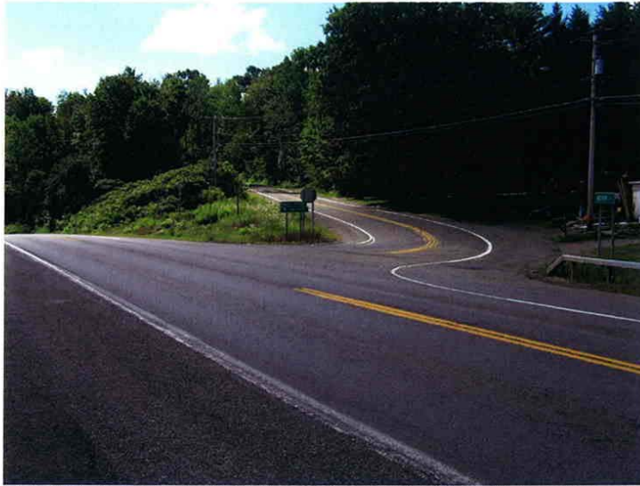
Photograph 29 Looking south at the intersection at Kimball Stand. There is a bridge over an unnamed tributary to Cassadaga Creek on the right side of the photograph.
