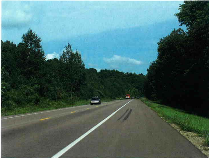
Photograph 9 Looking north on US Rt. 62, 2.5 miles north of the NY/PA boundary. There are two 11.5' wide lanes and 9' wide paved shoulders.
