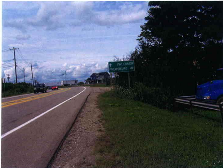
Photograph 11 Looking north on CR 380, at the intersection with CR 55.
