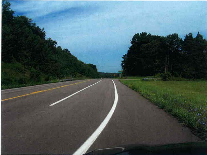
Photograph 3 Looking north on US Rt. 62, 0.5 miles north of the NY/PA boundary at Frissle Road. There are two 11.5' wide lanes, one 9' wide tuning lane and 5' wide paved shoulders.
