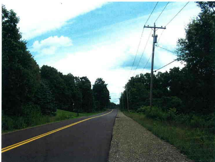
Photograph 8 Looking south on CR 65, 3.0 miles south of the intersection with NYS Rt. 60. There are two 11' wide lanes with 6.5' wide gravel shoulders.
