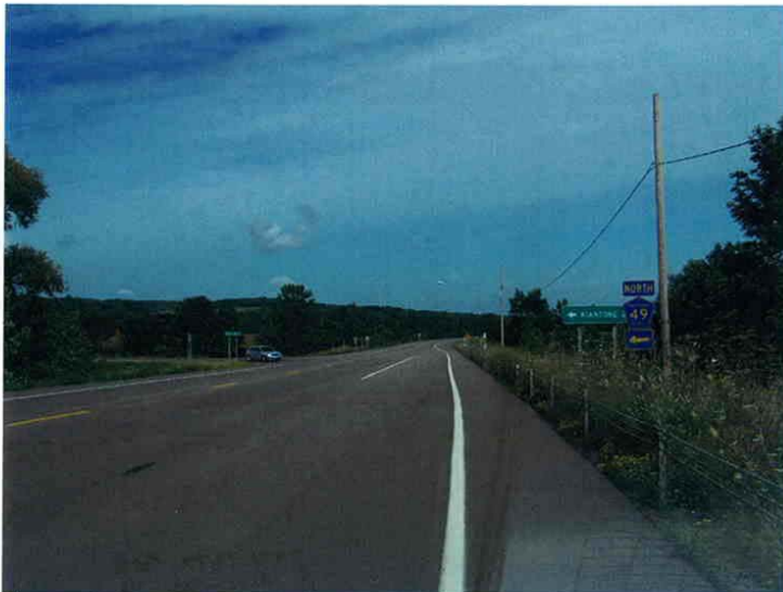
Photograph 4 Looking north on US Rt. 62, at the intersection of CR 49. There are two 11.5' wide lanes, one 9' wide tuning lane and 5' wide paved shoulders.
