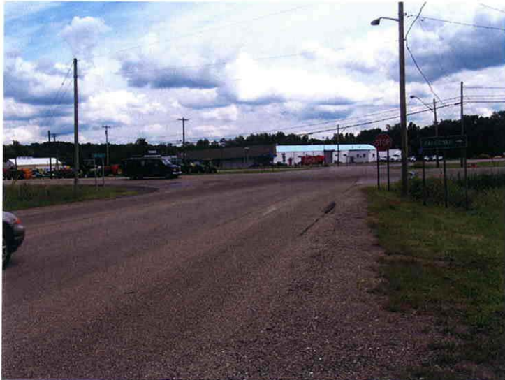
Photograph 13 Looking south on CR 65 at the intersection with NYS Rt. 395 at Levant. There are two 11' wide lanes with 6.5' wide gravel shoulders. Only traffic on CR 65 is required to stop at this intersection.
