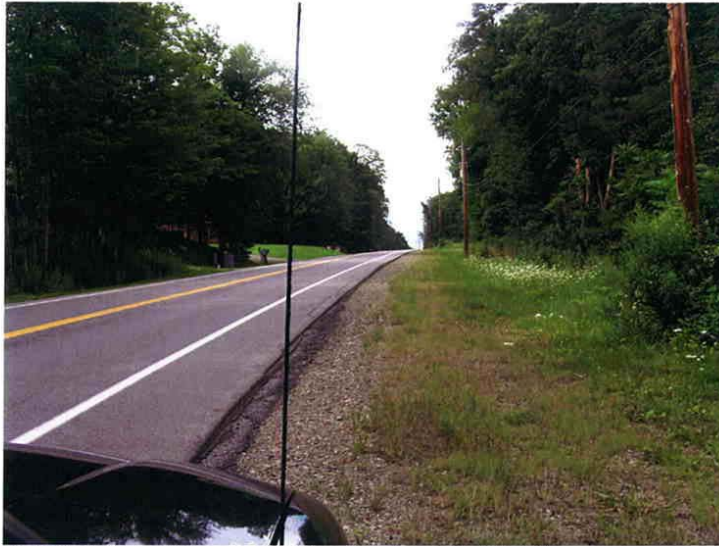
Photograph 21 Looking north on CR 380, 0.5 miles north of the I-86 overpass.
