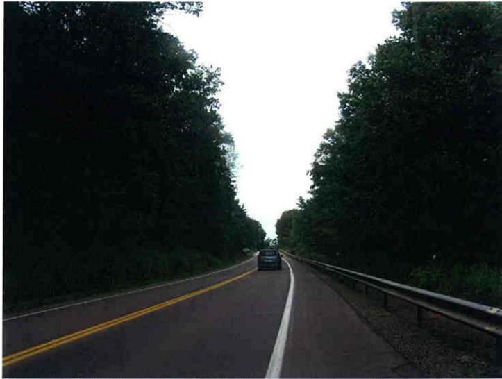
Photograph 23 Looking north on CR 380, 1.5 miles north of the I-86 overpass.
