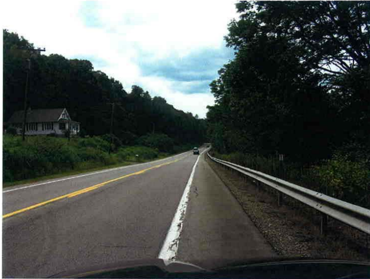
Photograph 25 Looking north on CR 380, 2.0 miles north of the I-86 overpass.
