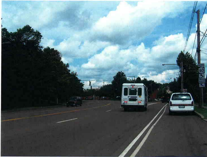
Photograph 11 Looking north on NYS Rt. 60 at the signalized intersection with Foote Avenue. There are four 13' wide lanes, a 15' wide lane and a 9' wide parking lanes. Note the sign identifying the road as a truck route.
