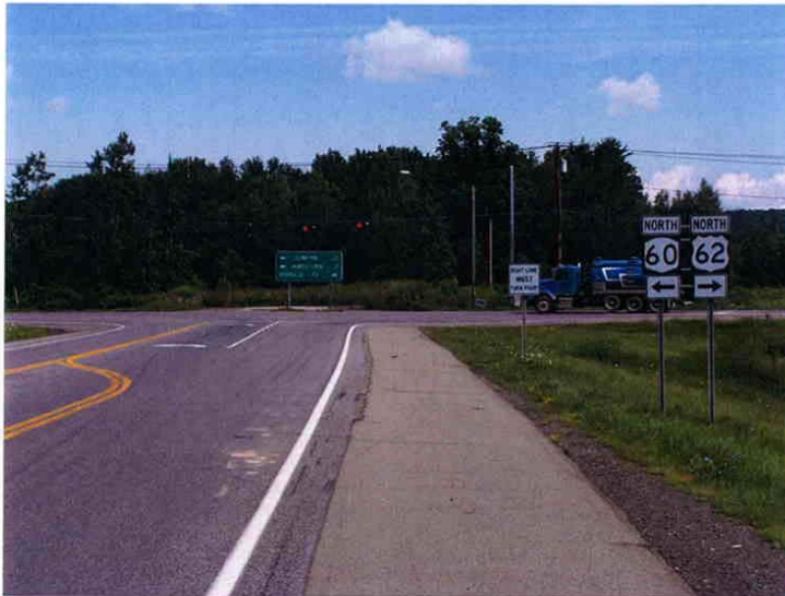
Photograph 14 Looking north on US Rt. 62 at the signalized intersection with NYS Rt. 60, 4.3 miles north of the NY/PA boundary. There are two 11.5' wide lanes and 9' wide turning lane and 5.5 wide paved shoulders. This is also the general area when a new segment of road is proposed.
