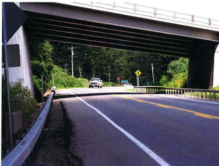
Photograph 28 Looking north at the NYS Rt. 60 overpass.
