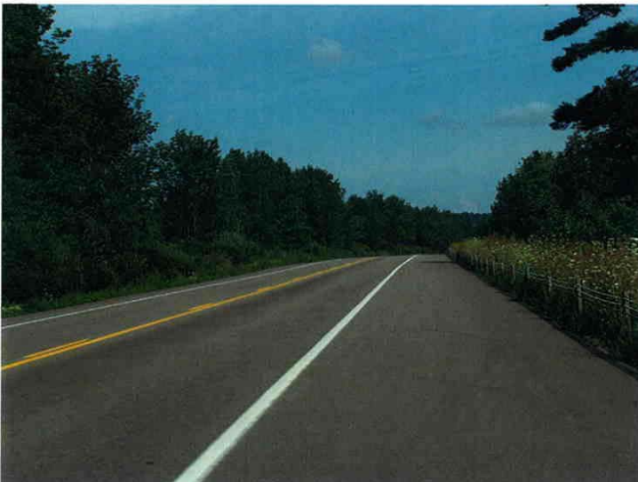
Photograph 10 Looking north on US Rt. 62, 3.0 miles north of the NY/PA boundary. There are two 11.5' wide lanes and 9' wide paved shoulders.
