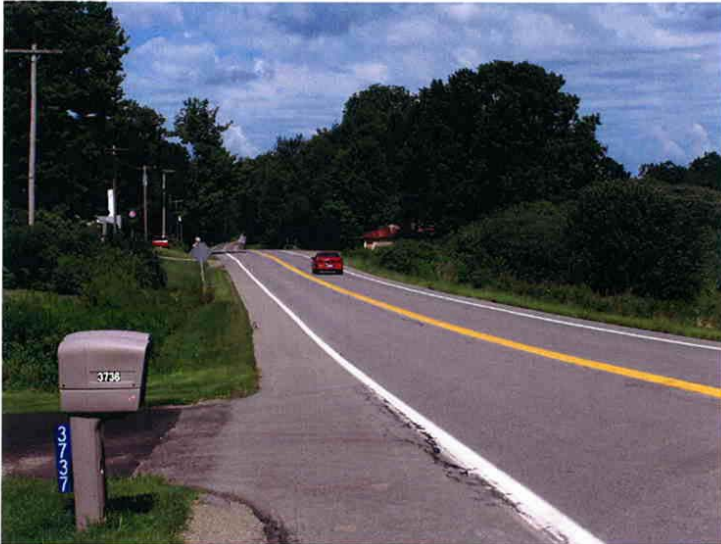
Photograph 26 Looking north on CR 380, 1.0 miles south of the NYS Rt. 60 overpass.
