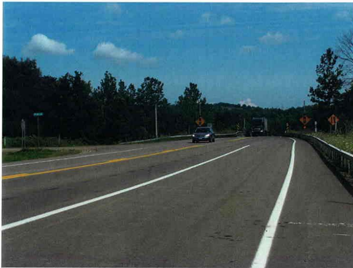
Photograph 12 Looking north on US Rt. 62, at the intersection with Spencer Road. There are two 11.5' wide lanes, a 9' wide passing lane and a 9' wide paved shoulders.
