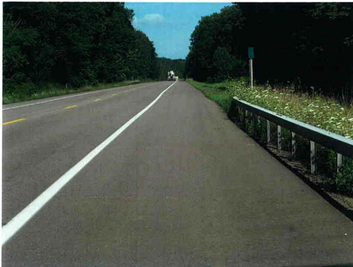
Photograph 8 Looking north on US Rt. 62, 2.0 miles north of the NY/PA boundary. There is a small culvert in the background. There are two 11.5' wide lanes and 9' wide paved shoulders.
