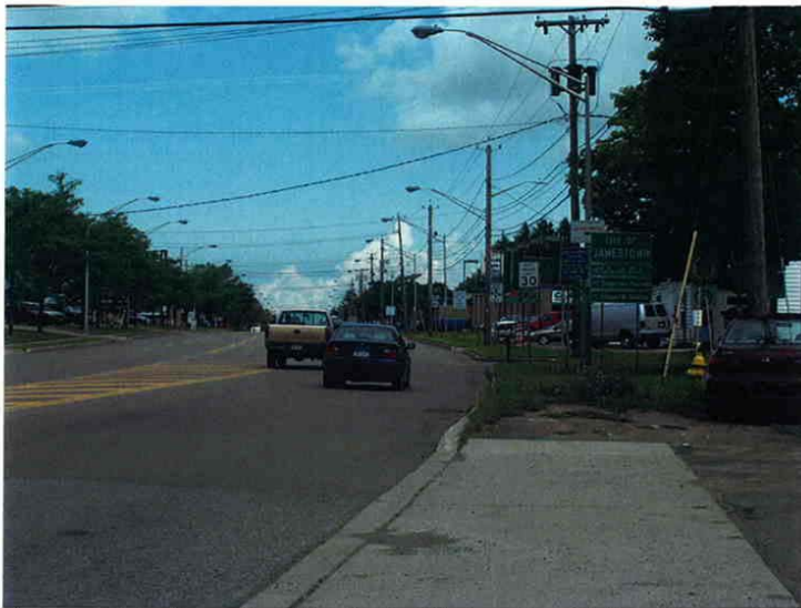
Photograph 8 Looking north on NYS Rt. 60, at the Jamestown City line. There are four 13' lanes and the speed drops to 30 mph.
