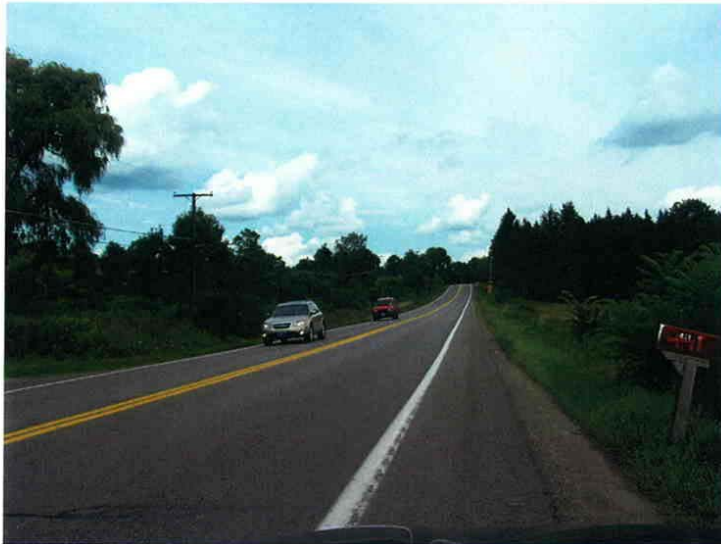
Photograph 5 Looking north on CR 380, 0.7 miles north of the intersection of CR 51 and NYS Rt. 60. There are two 11.5' wide lanes with a 3.5' wide paved shoulder throughout this section. The speed limit is 40 mph in this area.
