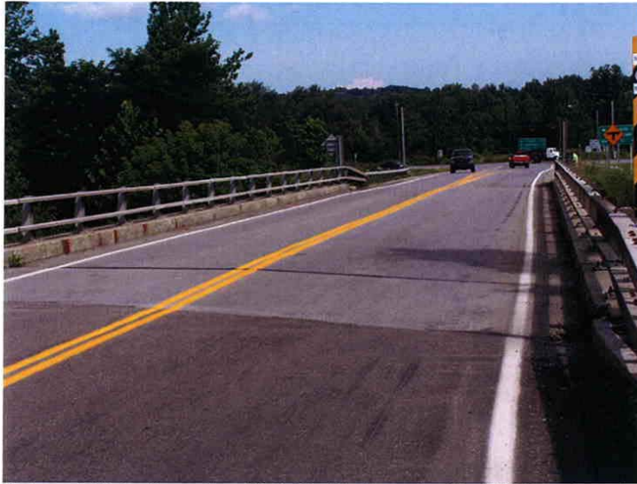
Photograph 13 Looking north on US Rt. 62, 4.3 miles north of the NY/PA boundary, at a bridge over Frew Run. There are two 11.5' wide lanes and 1.5' wide paved shoulders.
