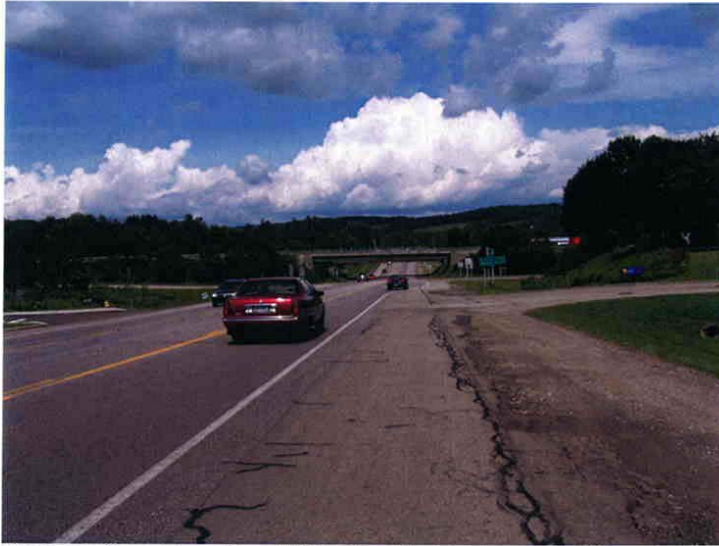
Photograph 29 Looking north on NYS Rt. 60 and the interchange with I-86.
