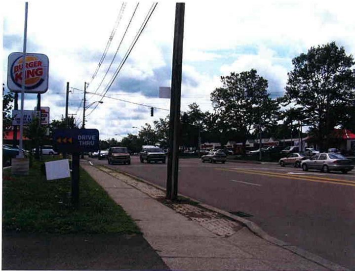
Photograph 9 Looking south on NYS Rt. 60 at the signalized intersection with Cole Avenue. There are four 13' wide lanes and a 9' wide turning lane.
