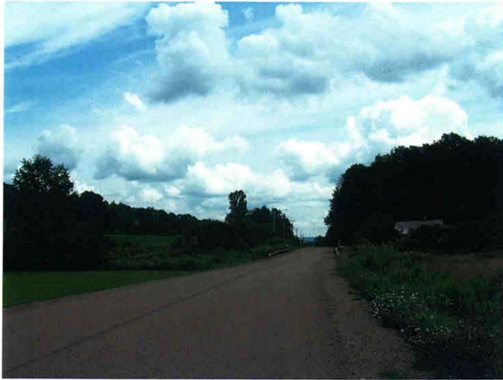
Photograph 11 Looking south on CR 65, 4.6 miles south of the intersection with NYS Rt. 60. There are two 11' wide lanes with 5' wide gravel shoulders.
