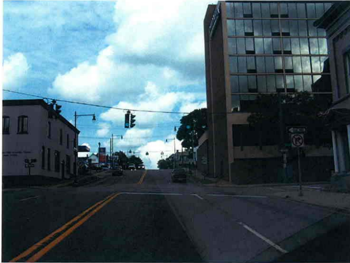
Photograph 17 Looking north on NYS Rt. 60 at the signalized intersection with West Fourth Street. There are four 13' wide lanes in this location.
