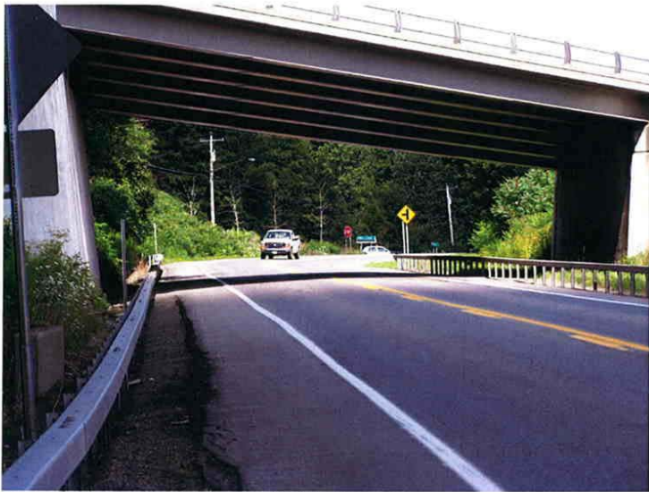
Photograph 28 Looking north at the NYS Rt. 60 overpass.
