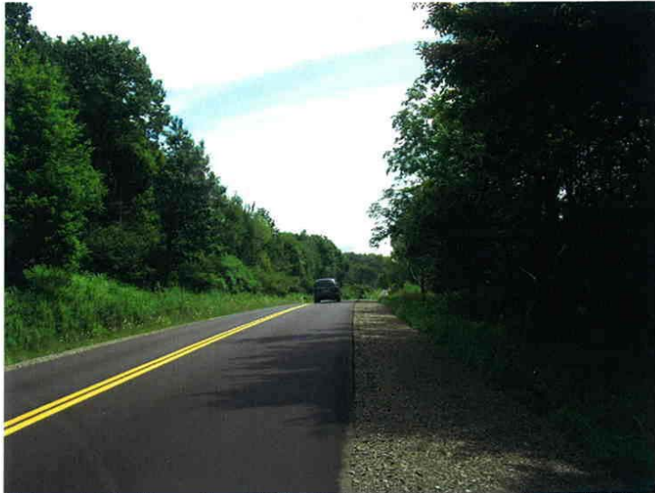
Photograph 3 Looking south on CR 65, 0.5 miles south of the intersection with NYS Rt. 60. There are two 11' wide lanes with 6.5' wide gravel shoulders.
