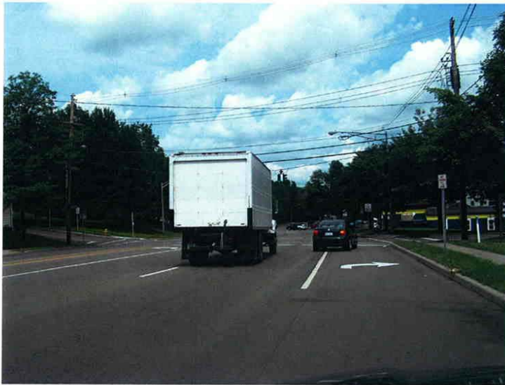
Photograph 10 Looking north on NYS Rt. 60 at the signalized intersection with Newland Avenue. There are four 13' wide lanes and two 9' wide turning lanes.
