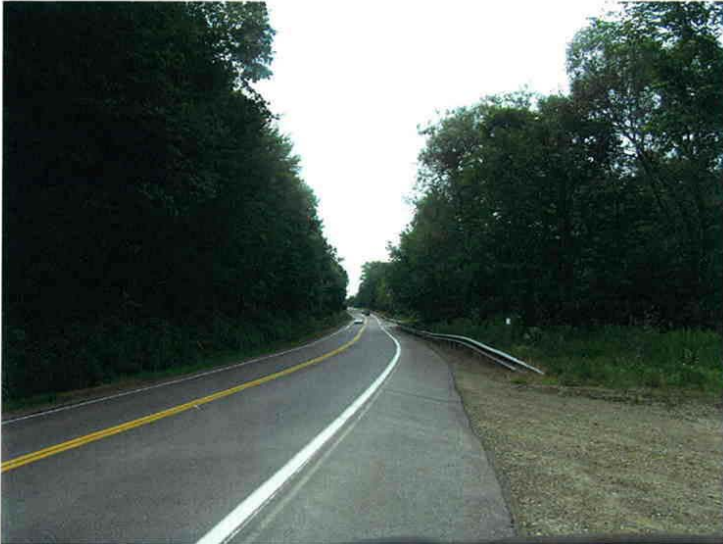
Photograph 24 Looking north on CR 380, 2.0 miles north of the I-86 overpass.
