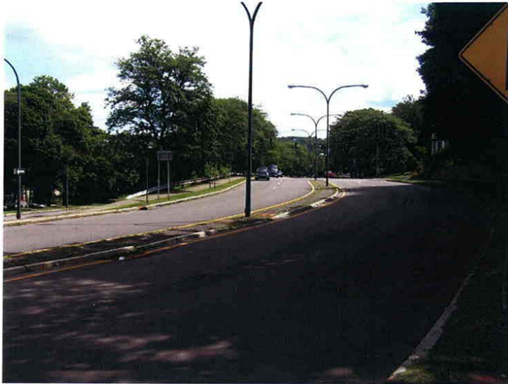
Photograph 13 Looking south on NYS Rt. 60 at the signalized intersection with Forest Avenue. This area transitions from four lanes to two lanes as the road approaches the Washington Street Bridge.
