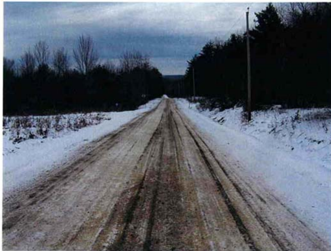
Photograph 18 Looking east on Swamp Road, past Seavert Road.
