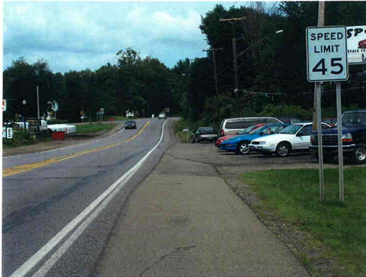
Photograph 5 Looking north on NYS Rt. 60, 1.0 miles north of the intersection with NYS Rt. 62. There are two 11.5' wide lanes and 5' wide paved shoulders.
