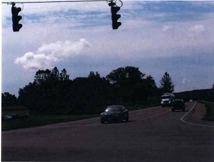
Photograph 1 Looking south across the intersection of NYS Rt. 60 and NYS Rt. 62.
