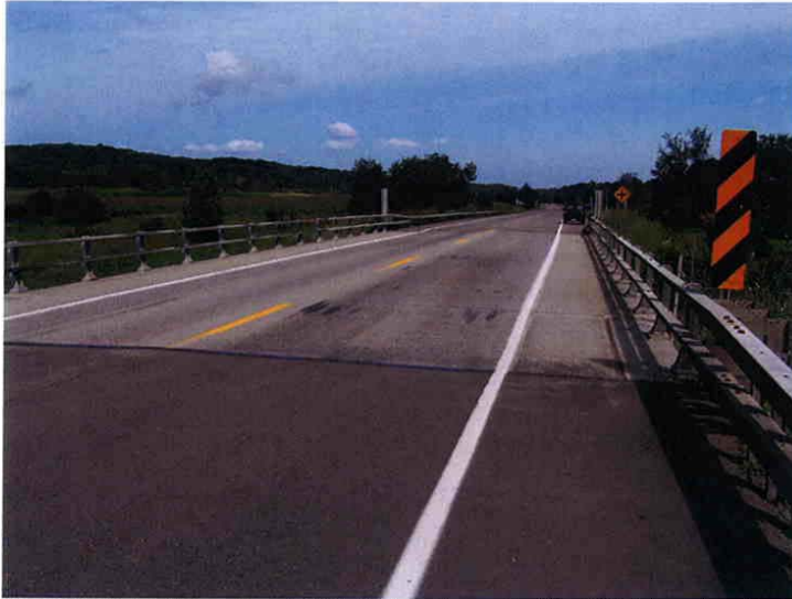
Photograph 5 Looking north on US Rt. 62, 1.0 miles north of the NY/PA boundary at a bridge over Kiantone Creek. There are two 11.5' wide lanes and 5' wide paved shoulders.
