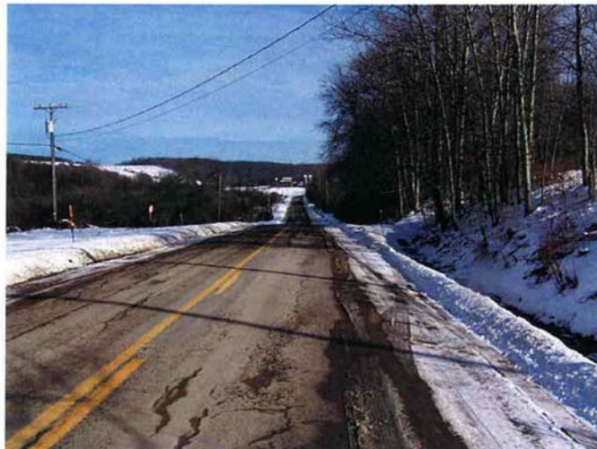
Photograph 4 County Road 46, 2.0 miles east of the Village of Franklinville.
