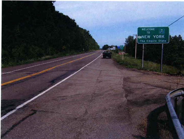
Photograph 2 Looking north at US Rt. 62. There are two 11.5' wide lanes with 9' wide paved shoulders.
