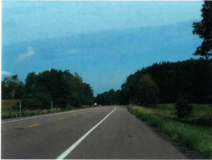
Photograph 7 Looking north on US Rt. 62, 1.5 miles north of the NY/PA boundary. There are two 11.5' wide lanes and 9' wide paved shoulders.
