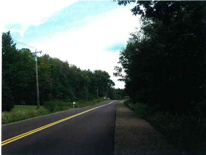
Photograph 9 Looking south on CR 65, 3.5 miles south of the intersection with NYS Rt. 60. There are two 11' wide lanes with 6.5' wide gravel shoulders.
