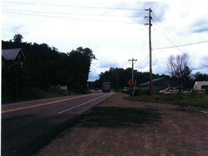
Photograph 20 Looking north on CR 380. The roadway has two 11.5' wide lanes and 4' wide shoulder in this area.
