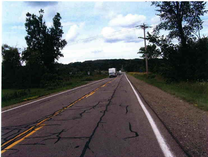
Photograph 2 Looking north along CR 51. There are two 12' wide lanes and 5' wide gravel shoulders throughout this segment. The speed limit is not posted on this segment.
