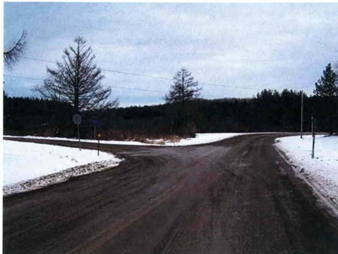
Photograph 26 The intersection of Allegany County Route 16 and Allegany County Route 15A.
