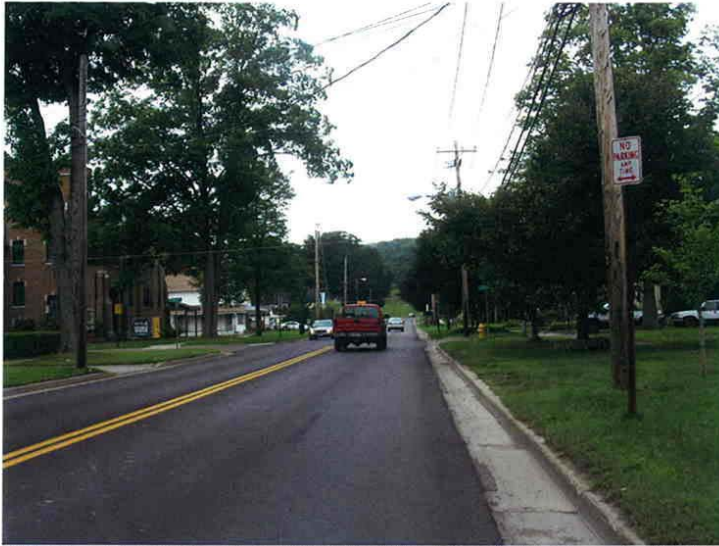
Photograph 17 Looking north on CR 380 (North Work Street), 0.2 miles north of the intersection with NYS Rt. 394. This section through the Village of Falconer has two 13' wide lanes and a concrete shoulder.
