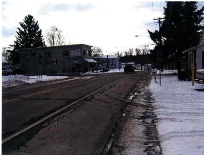
Photograph 11 New York State Route 19 and the intersection with Allegany County Route 46 in the hamlet of Caneadea.
