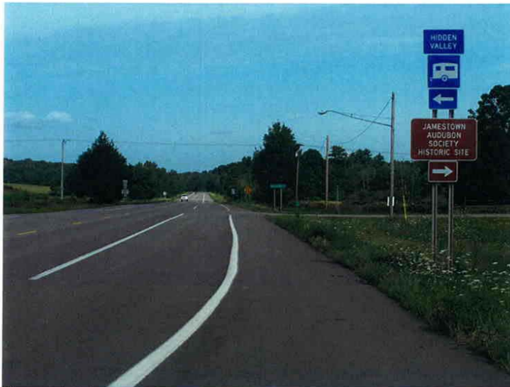
Photograph 6 Looking north on US Rt. 62, 1.1 miles north of the NY/PA boundary at Riverside Drive. Road. There are two 11.5' wide lanes, one 9' wide tuning lane and 5' wide paved shoulders.
