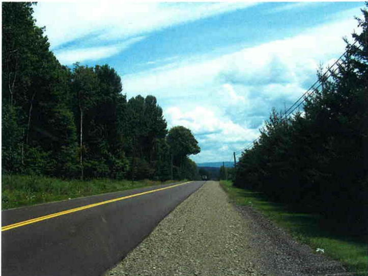
Photograph 4 Looking south on CR 65, 1.0 miles south of the intersection with NYS Rt. 60. There are two 11' wide lanes with 6.5' wide gravel shoulders.
