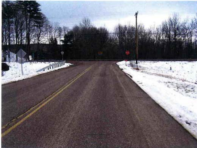
Photograph 5 The intersection of Allegany County Routes 16 and 15.
