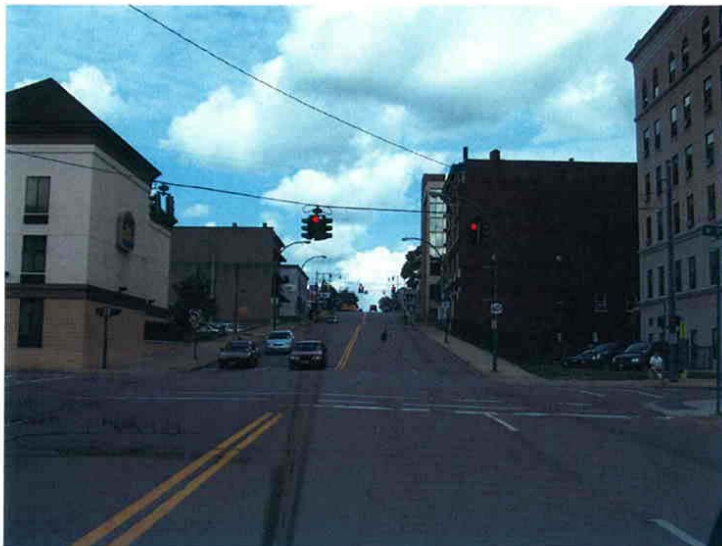
Photograph 16 Looking north on NYS Rt. 60 at the signalized intersection with West Third Street. There are four 13' wide lanes in this location.
