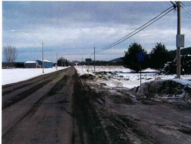
Photograph 6 Allegheny County Route 7B at Hardy Corners.
