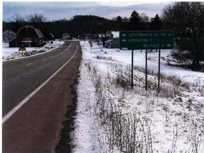
Photograph 10 NYS Route 243 and its intersection with New York State Route 19.
