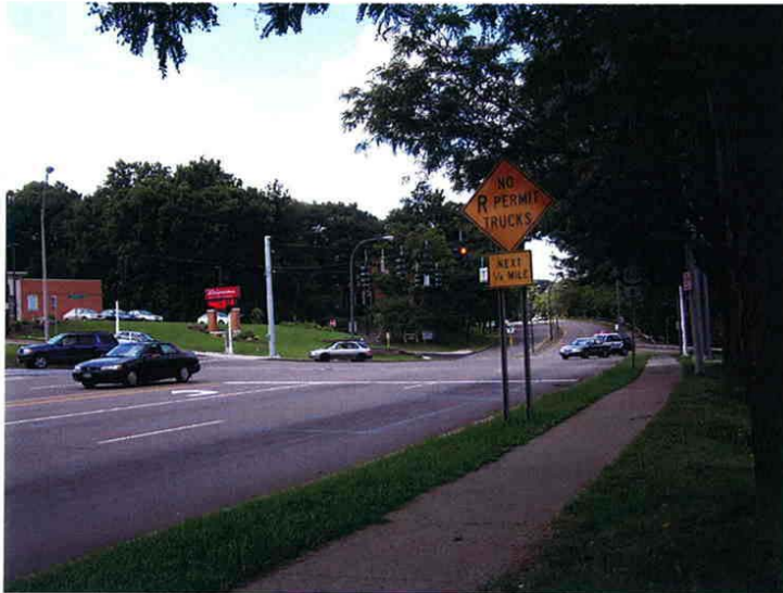
Photograph 12 Looking north on NYS Rt. 60 at the signalized intersection with Main Street. There are four 13' wide lanes and a 9' wide turning lane.
