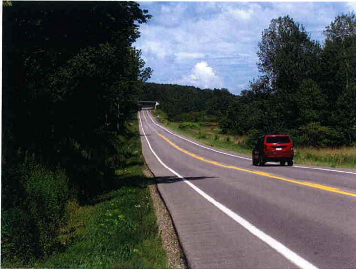
Photograph 27 Looking north on CR 380, 0.5 miles south of the NYS Rt. 60 overpass.
