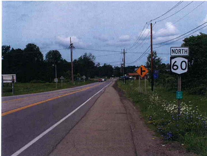
Photograph 2 Looking north at NYS Rt. 60, 0.1 miles north of intersection with NYS Rt. 62. There are two 11.5' wide lanes with 6' wide paved shoulders. The speed limit is unmarked in the area.
