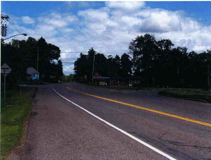
Photograph 30 Looking north on CR 380 at the intersection with CR 44 (Salisbury Road). With exception of northbound to NYS Rt. 60, all traffic must stop at this intersection.
