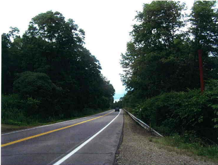
Photograph 22 Looking north on CR 380, 1.0 miles north of the I-86 overpass.
