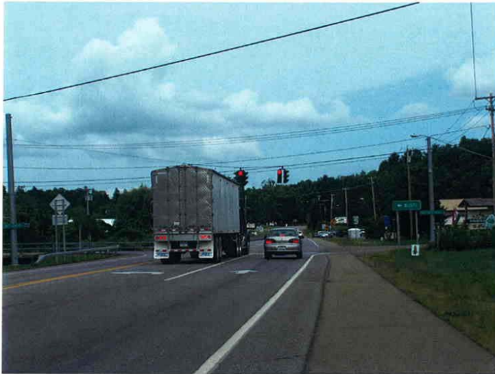
Photograph 4 Looking north on NYS Rt. 60, at the signalized intersection of CR 380 (Peck Settlement Road). There are two 11.5' wide lanes, one 9' wide tuning lane and 7' wide paved shoulders.
