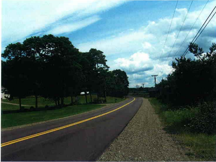
Photograph 5 Looking south on CR 65, 1.8 miles south of the intersection with NYS Rt. 60. There are two 11' wide lanes with 6.5' wide gravel shoulders.
