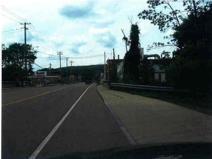
Photograph 15 Looking north at the bridge over the Chadakoin River. There are two 11.5' wide travel lanes and a 6.0 wide paved shoulder.
