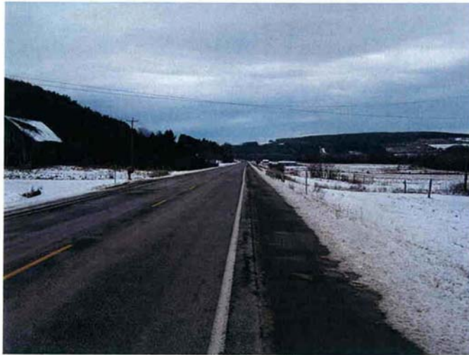
Photograph 30 NYS Route 70 east of the intersection with Allegheny County Route 15.
