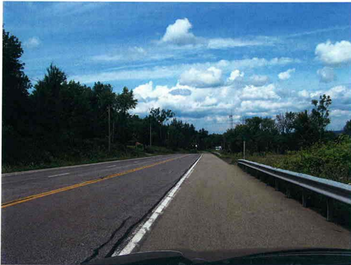
Photograph 34 Looking north on NYS Rt. 60 where it is a three-lane.
