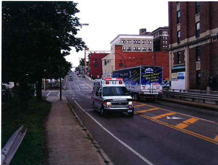
Photograph 15 Looking north on NYS Rt. 60 (Washington Street) at the signalized intersection with West Second Street. There are two 13' wide lanes and one 2' wide shoulder.
